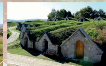
Köporos wine cellars built walkways and lightning.
